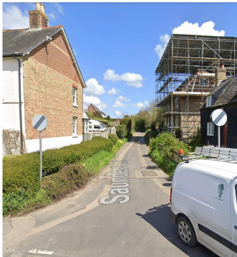
Figure 2: View of Saunders Lane from New Street looking north (courtesy of Google dated April 2023)
