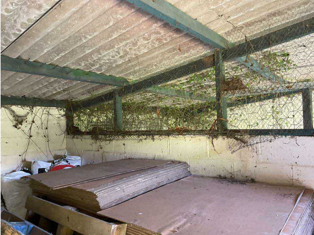
View of interior of stables showing timber purlin roof over stored materials
