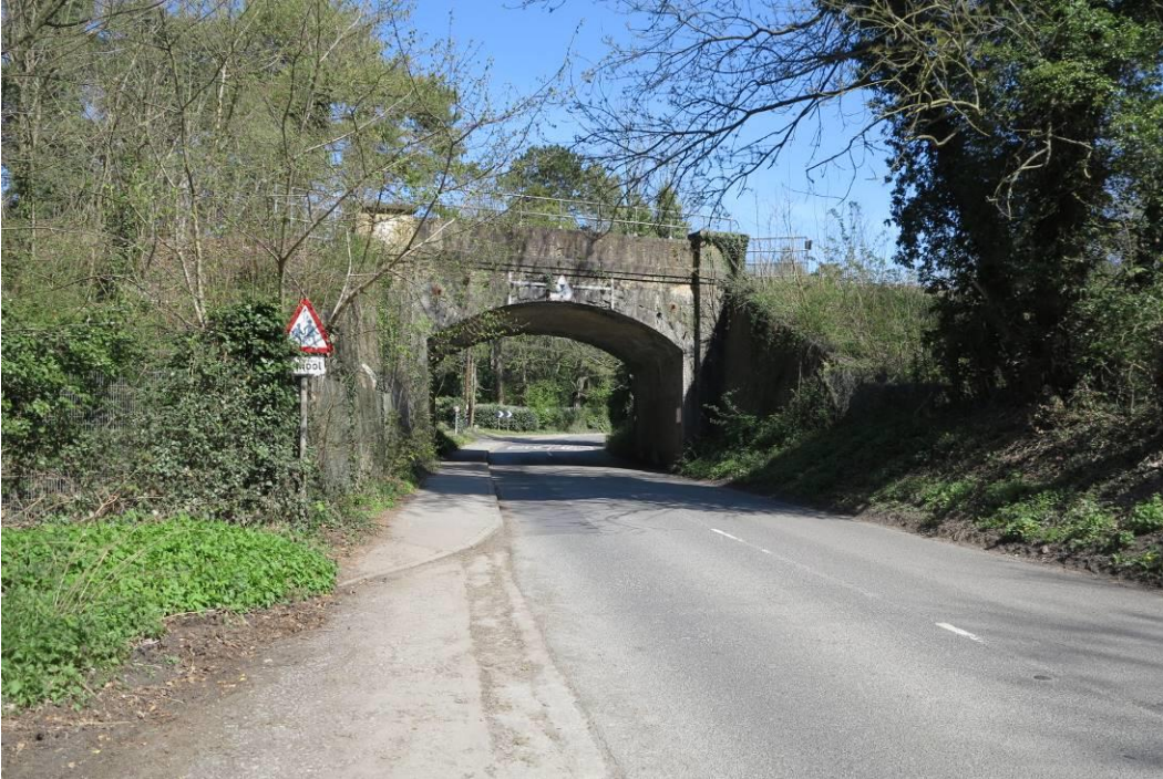
Plate 1. Looking towards the railway bridge from the south-west
