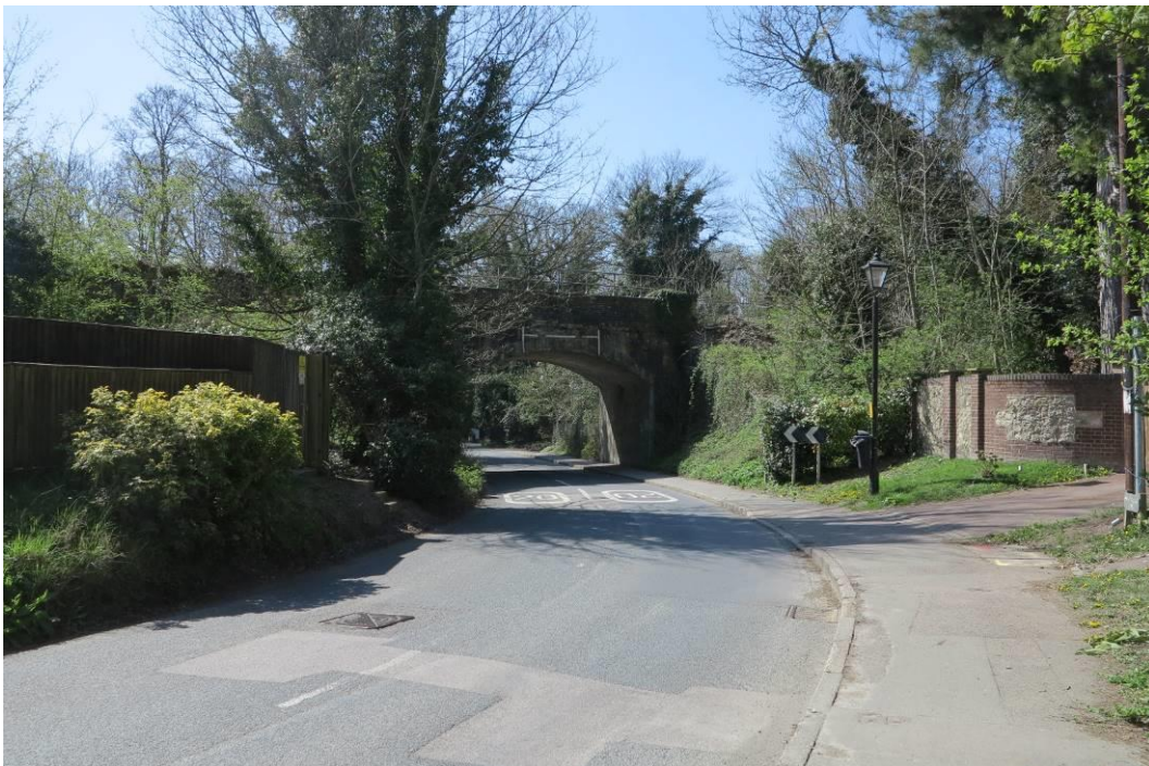
Plate 2. Looking towards the railway bridge from the east
