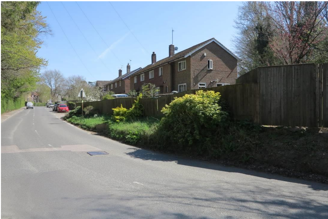
Plate 30. 20 th -century housing on Eyhorne Street beyond the railway bridge
