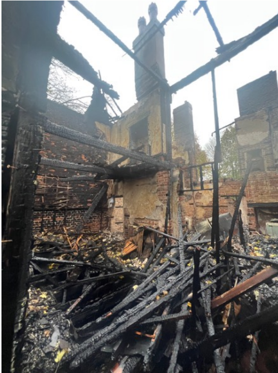
The partially suspended ground floor, first floor, and roof structure have been lost.
