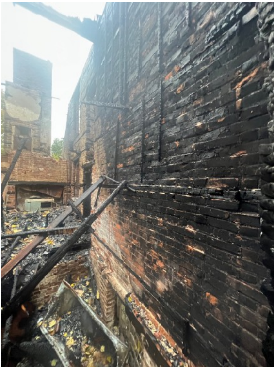
The floor plates and timber lintels built into the external walls have been damaged or lost.
