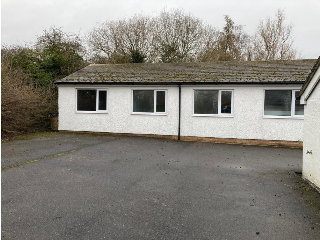
The roof coverings appear to be modern asbestos slate on the north shed.
