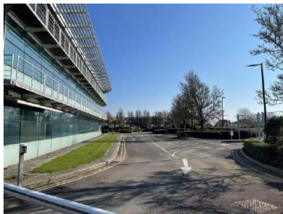
View to the site entrance of hardstanding, amenity grassland, building 1 and introduced shrub.
