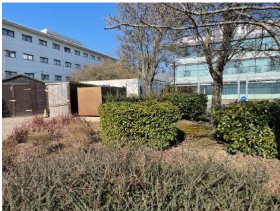
View of buildings 1, 2, 3, 4 and 5 and introduced shrub.
