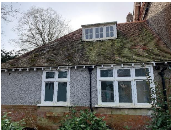
Plate 17. Several missing roof tiles on the eastern extension of B1.
