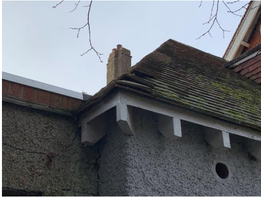
Plate 15. Lifted hip tiles providing bat roost potential on the eastern extension of B1
