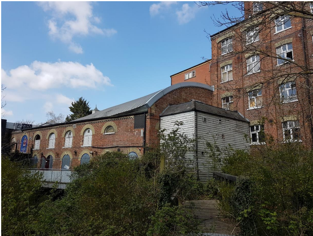
Plate 25. Wooden bridge providing access over the East Stour River to the separate island in the northeast of the Site.
