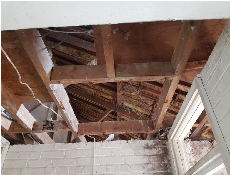
Plate 1. B1- High suitability to support roosting bats, internal view. Gaps under remaining insulation and between insulation and timber frame.
