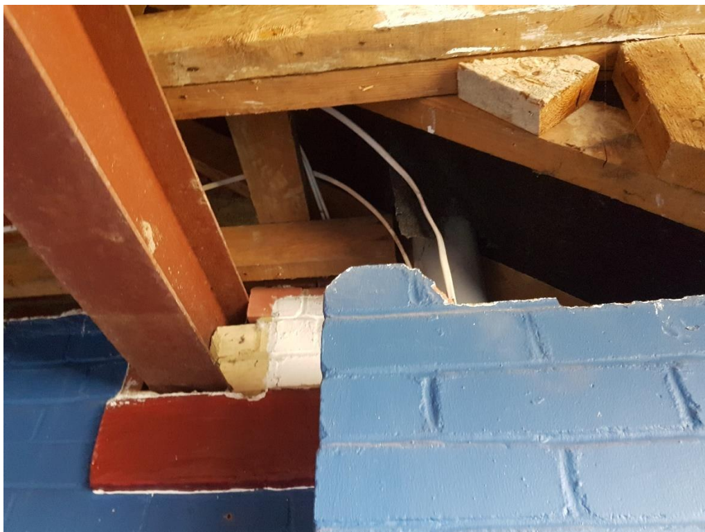
Plate 6. B1- High suitability to support roosting bats, internal view. Cavities in walls leading into the roof.
