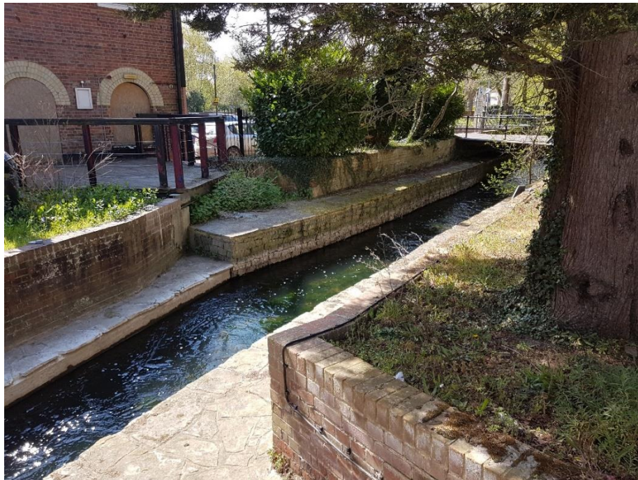
Plate 16: The Great Stour, runs along the western boundary of the Site in a northerly direction. Access to the building (B1) on Site is provided by two bridges across the river.
