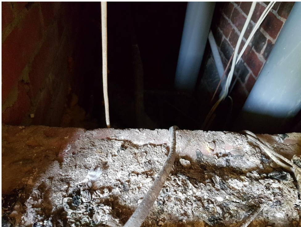
Plate 2. B1- High suitability to support roosting bats, internal view. Cavities present in and behind walls, blocked from sunlight.
