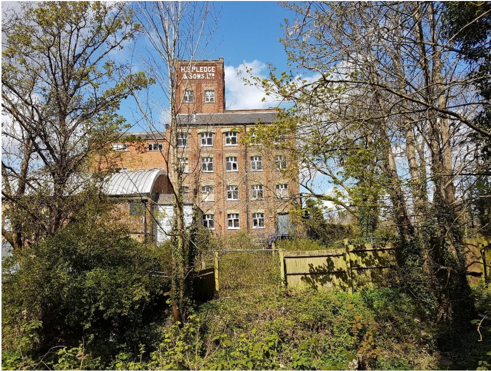
Plate 24. Building, view from footpath (outside of the Site boundary). Image of inaccessible area (southeast of Site) due to overgrown vegetation.
