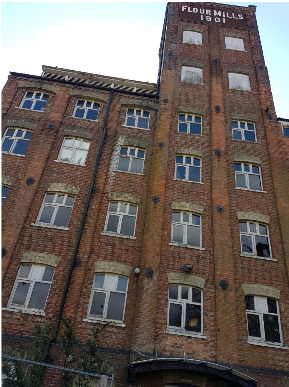
Plate 13. B1- High suitability to support roosting bats, external view. Multiple broken windows throughout the building. The top two floors of the tower are inaccessible. The majority of the building is five-storeys, with the tower adding an additional two storeys.
