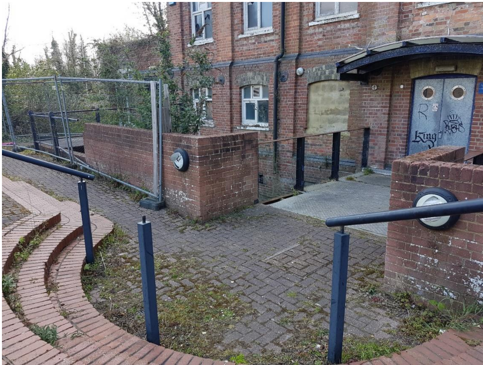
Plate 15. Hardstanding in front of the building (B1) in the west of the Site. Bridge over the river provides original access to the building (currently inaccessible through the pictured doorway).
