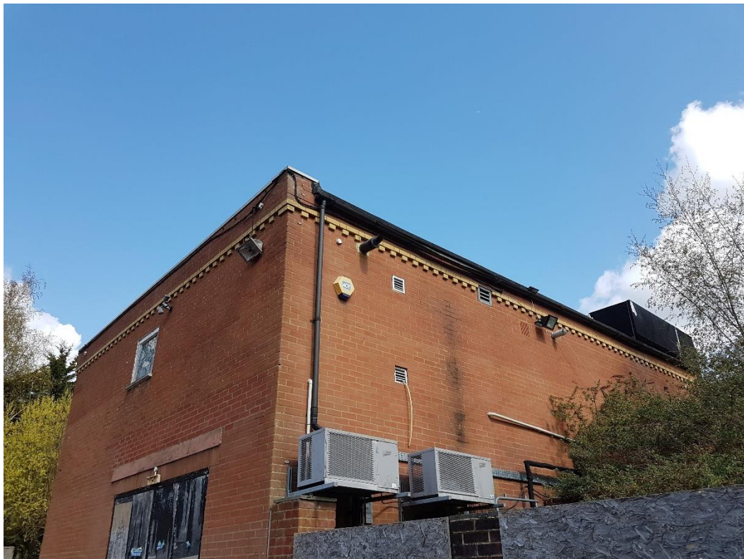
Plate 10. B1- High suitability to support roosting bats, external view. Potential access through vents along the southeast of the building.
