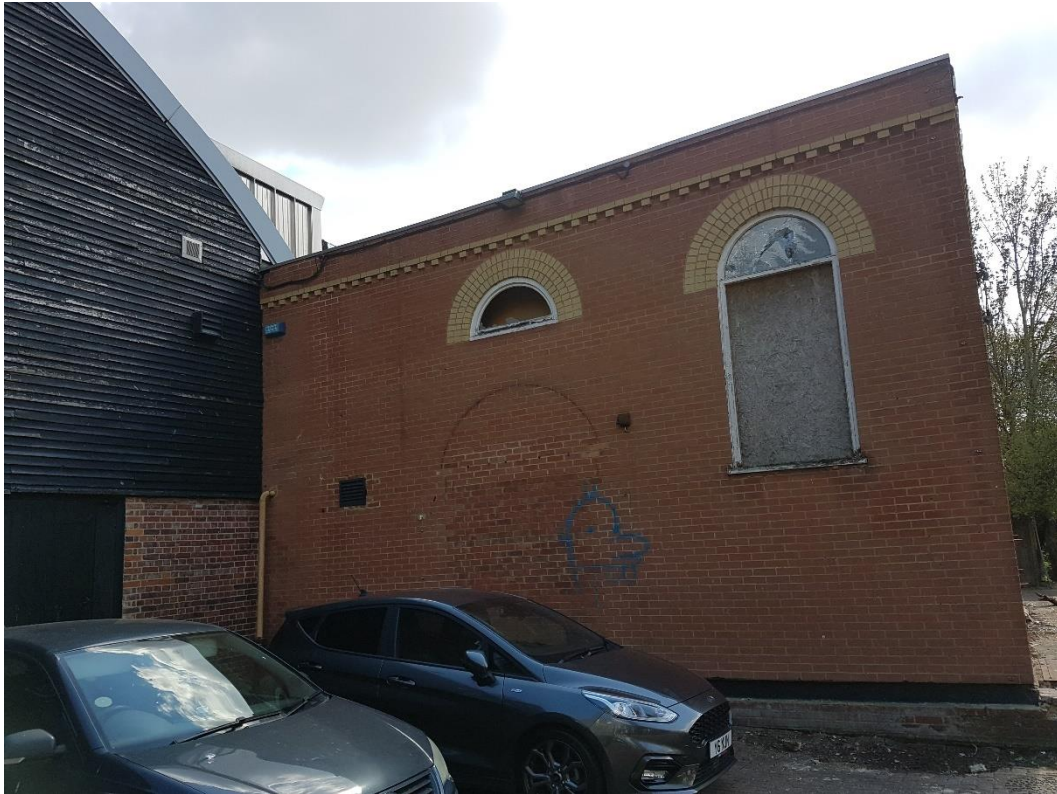
Plate 11. B1- High suitability to support roosting bats, external view. Broken windows and potential access through vents facing south west.
