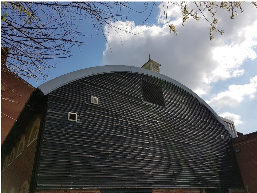
Plate 12. B1- High suitability to support roosting bats, external view. Large vent and ventilation tower on the roof of the southeastern section of the building. Ventilation tower faces to the southwest.
