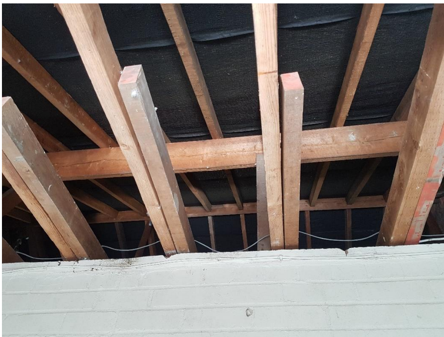
Plate 4. B1- High suitability to support roosting bats, internal view. Gaps between bitumen felt lining and timber frame and gaps underneath internal felt lining.
