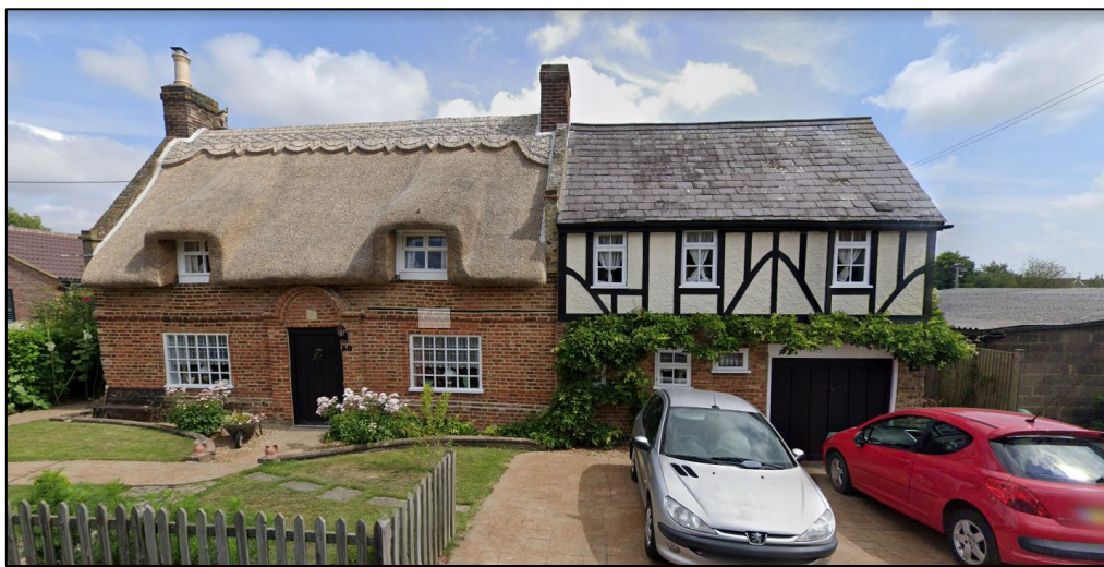
No. 50 New Street (Courtesy Google Maps Streetview)
