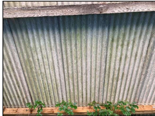
Plate 22.. Potential ACM present on the rooves of the buildings in the south of the Site.
