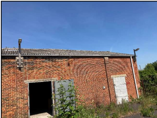
Plate 21. Potential ACM present on the rooves of the buildings in the south of the Site.
