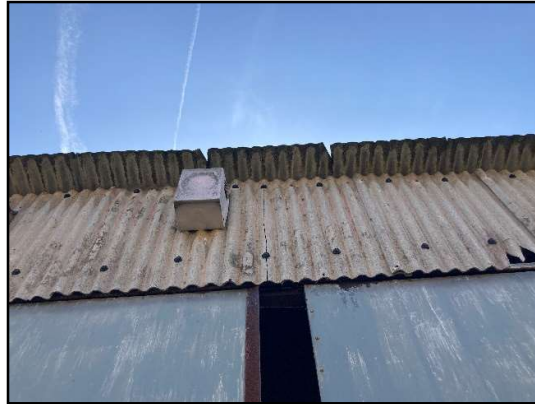
Plate 20.. Potential ACM present on the rooves of the buildings in the south of the Site.
