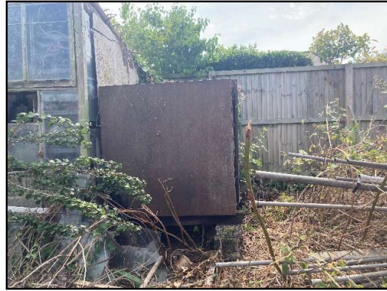
Plate 14.. AST raised on bricks present adjacent to the greenhouse in the southwest of the Site.
