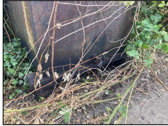
Plate 16.. Unbundled AST present adjacent to the gate (Plate 1), some evidence of staining noted.
