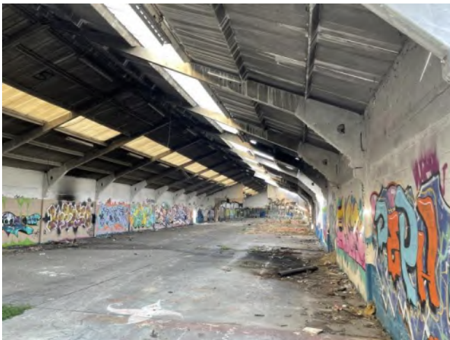
Photo 15: Inside southern building, with corrugated ACM internal roofing and concrete floor (looking west)
