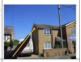
Workshop B is single skin brick and corrugated fibre cement roof sheets. But there is a gap leading under the ridge tiles.
