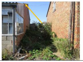
The large workshop C is single skin brick and corrugated fibre cement roof sheets. But there are gaps leading under the ridge
