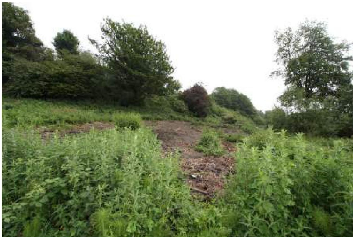
View of Site from Romney Avenue prior to fill placement 30 th May 2018
