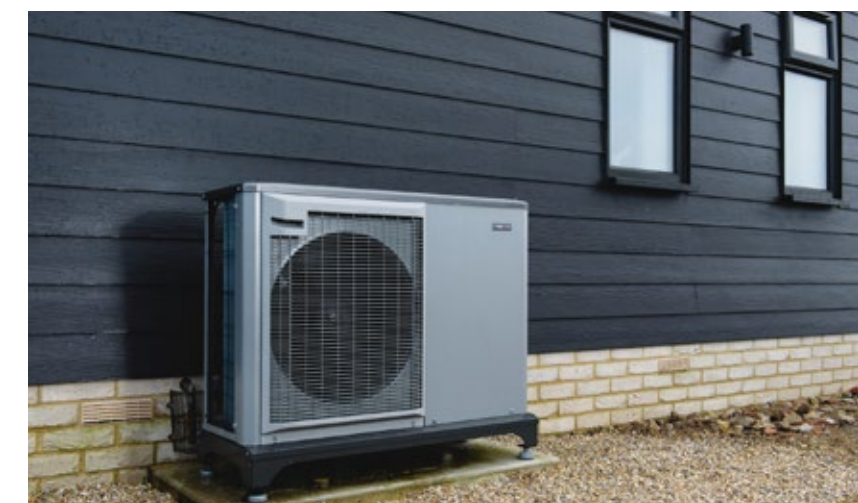
Air source heating unit
