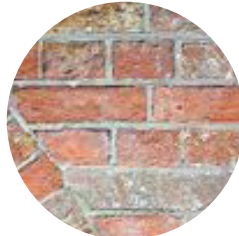
RED MULTISTOCK BRICK OF EXISTING FLOUR MILL
