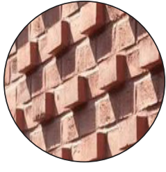
RECESSED BRICKWORK DETAIL
