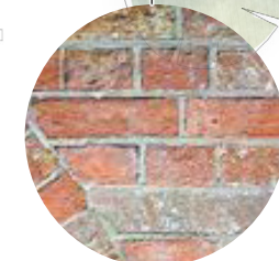
RED MULTISTOCK BRICK TO EXISTING FLOUR MILL
