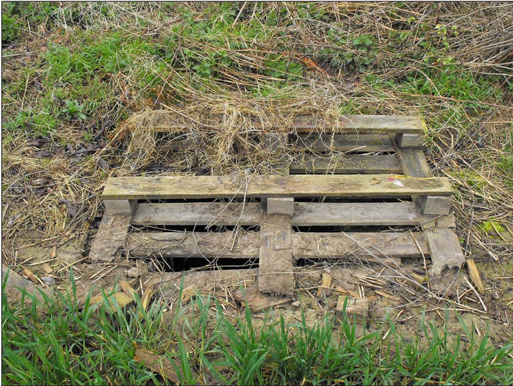
Plate 2. Deep void, possibly brick lined well, covered by wooden pallet along western edge of site. View facing west.
