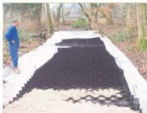
Cellweb during installation.
