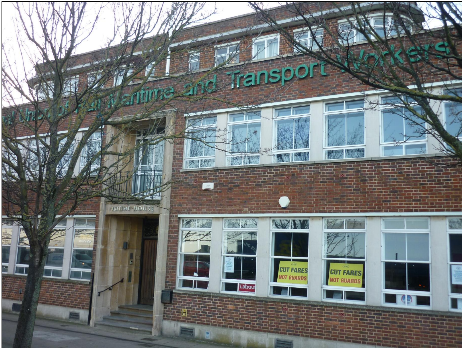
Figure 3. The offices to the south.
