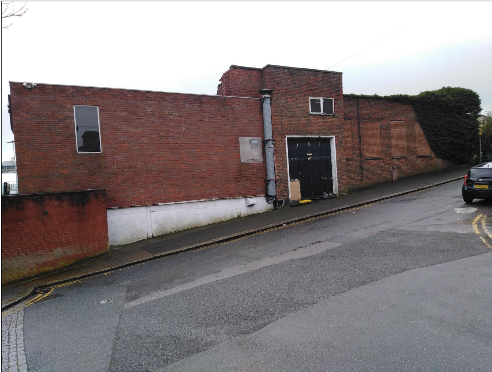
Figure 1. The building on the western part of the site
