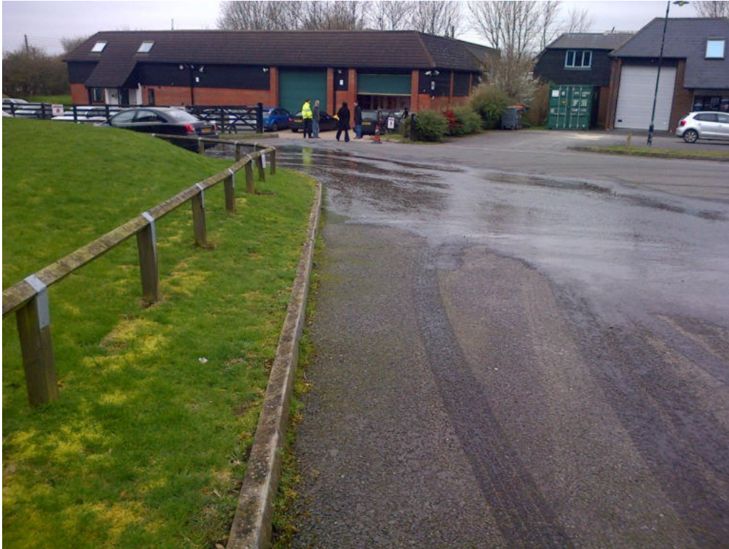
Groundwater flows issuing from overflowing soakaway at Northdown Close. Taken on 7 th March 2014 (Source: A. Brauningner, KCC)
