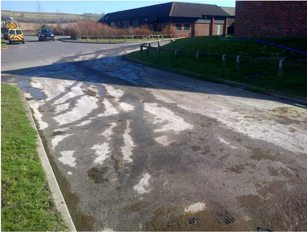
Excess groundwater flows alleviated by overpumping from soakaway into nearby highway culvert by landowner. Taken on 20 th March 2014. (Source: A Brauning, KCC)
