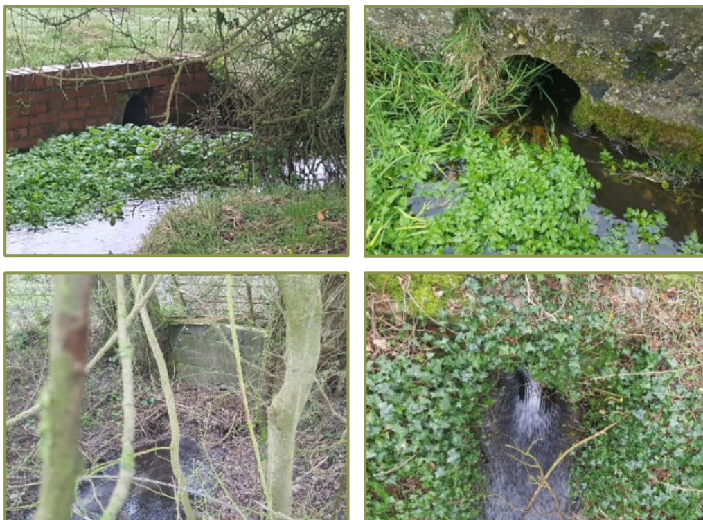
Top left: Ø300mm culvert outfalling into Watercourse 1. Top Right: Ø300mm culvert conveying flow beneath farm access track along Watercourse 1. Bottom left: Ø600mm culvert inlet into Watercourse 3. Bottom Right: Ø600mm culvert outfall into Watercourse 3.
